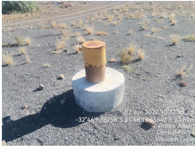
Monitoring Borehole
