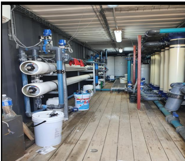
Reverse Osmosis and Ultra Filtration Plant
