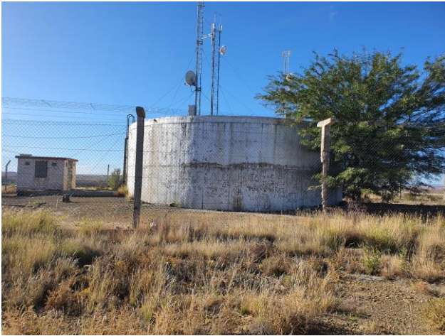
Raw water Storage Reservoir
